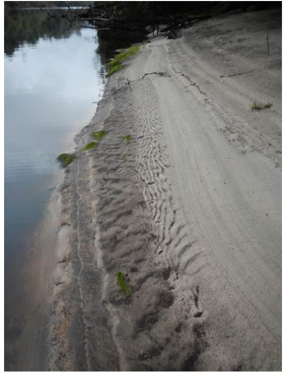
Figure 3-16: Mud veneers, ripple marks and recent scour on bank toe at erosion pin site 3C (zone 3).
