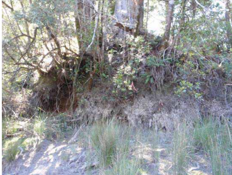
Photo 4-7 Erosion pin site 2G showing vegetation on bank in power station-controlled operating level, and collapse of root mat on left side of photo
