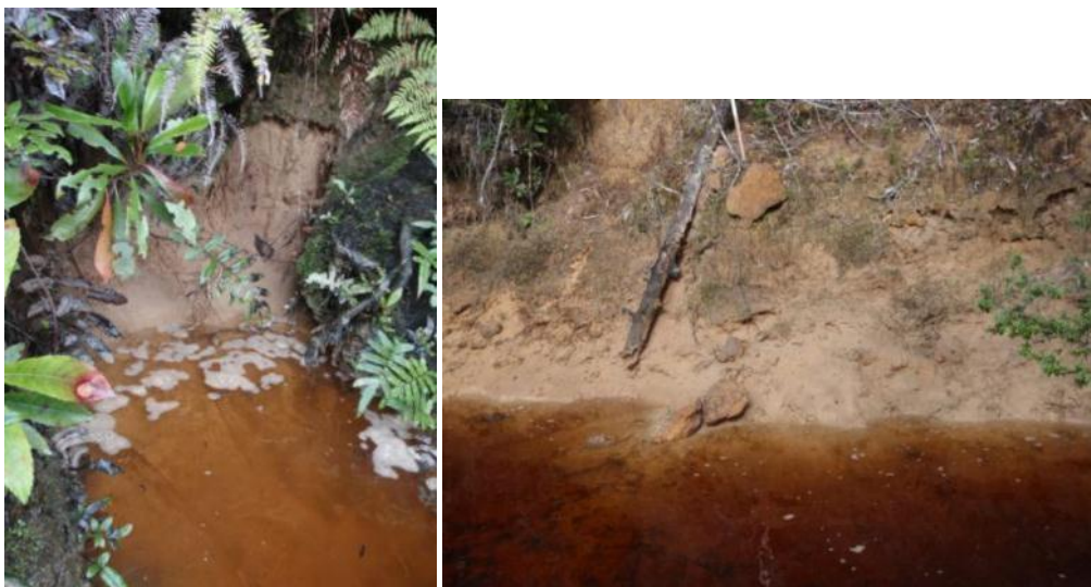
Photo A5-3 Exposed sands in 3-turbine bank level
