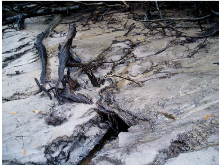
Photo 4.2. Bank erosion in zone 1 during high rainfall.
