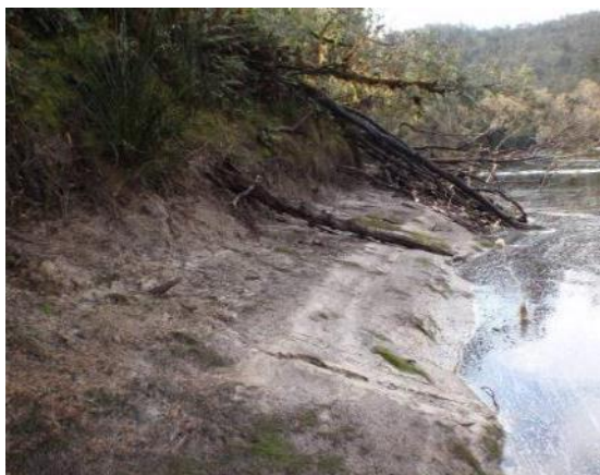
Photo 4-5 Break in slope at 2-turbine discharge level in zone 2 upstream of site 2C. Toe affected by seepage processes
