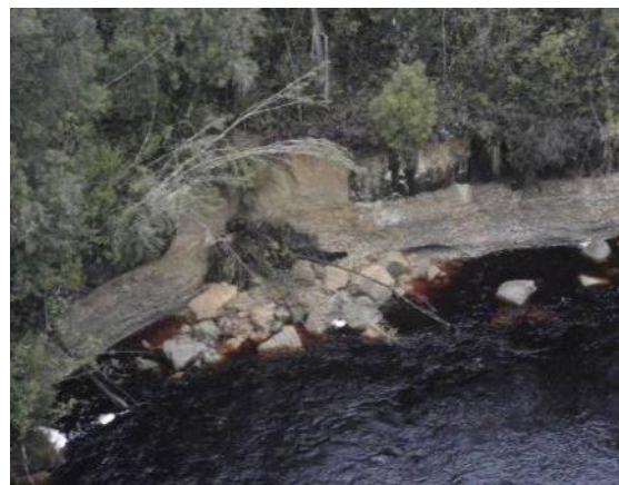
Photo 4-6 Bank failure on the left bank of lower Albert River
