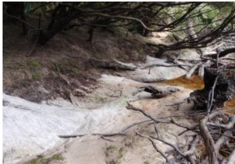
Photo 4-9 Sediment fans deposited at base of root mat. Sediment derived from seepage process
