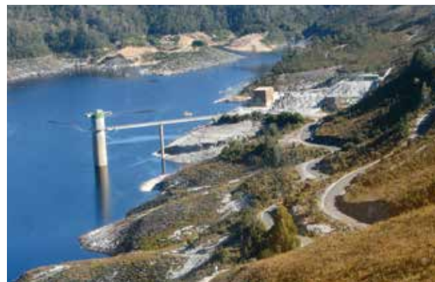
Gordon Power Station and its intake tower
