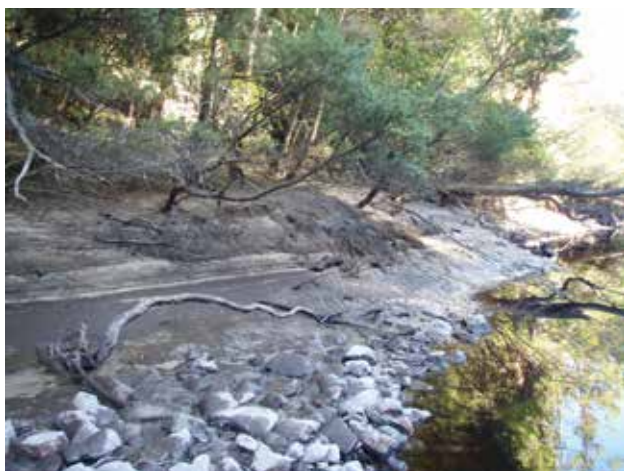
Bank erosion in zone 3
