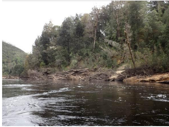
P4 – 2: Landslip at Denison confluence, October 2014
