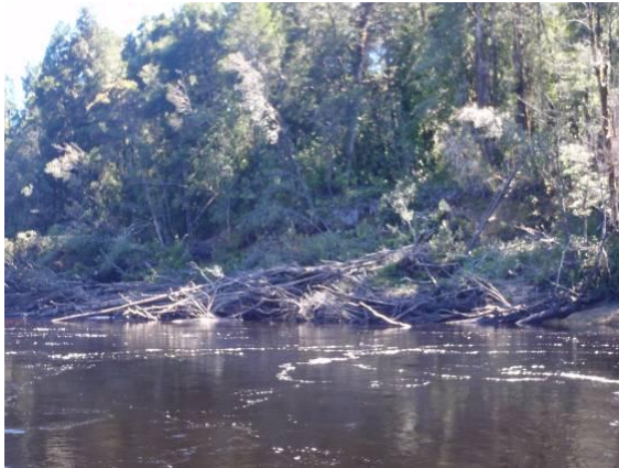
P4 – 2: Landslip at Denison confluence, October 2013
