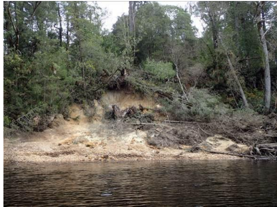
P2 - 5, zone 2, Landslip (previously P2 new1), October 2014
