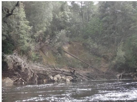
P4 – 1: Landslip at Denison confluence October 2014
