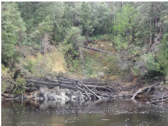
P4 – 1: Landslip at Denison confluence November 2013
