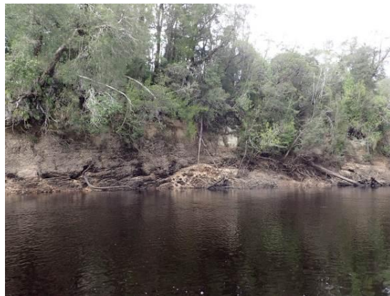
P2 - 8: Left Bank – close up of P2-7, October 2014 (not obtained in March 2014)
