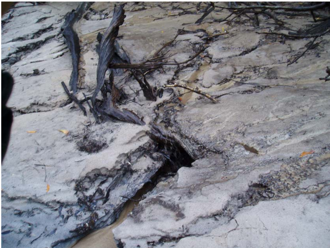
Photo 12.1. Erosion of exposed bank in zone 1 by rainfall during power station shut-down. Sediment is being transport by sheetwash and through rills. Deposition occurs at water level, as shown in next photo.
