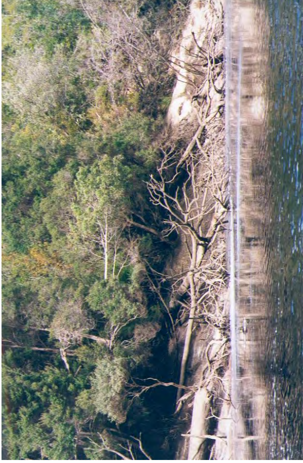
Photo 11. Alluvial bank with slots, voids
