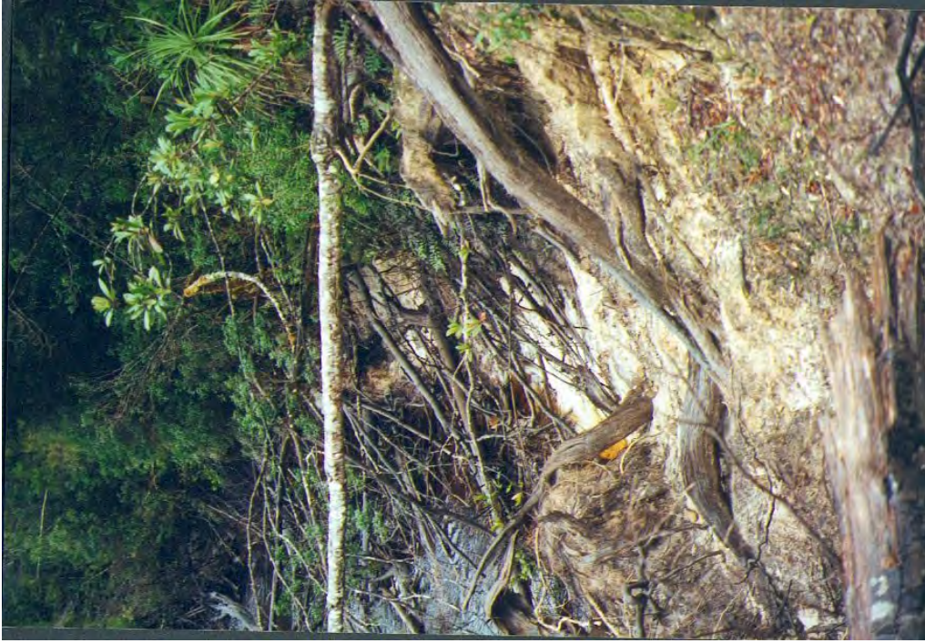
Photo 22. Undercutting of Albert River banks near mouth
