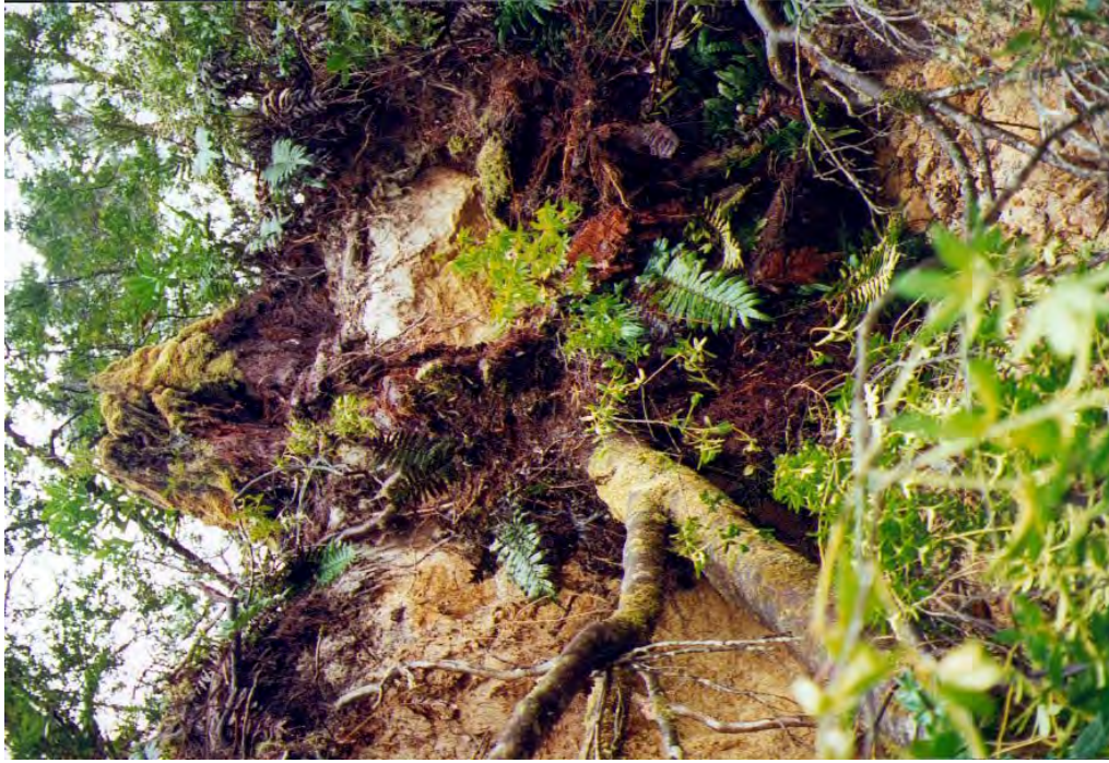
Photo 18. Additional tree fall in scarp in Zone 2
