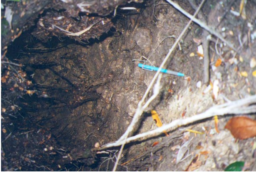
Photo 68. Exposed roots in undercut bank
