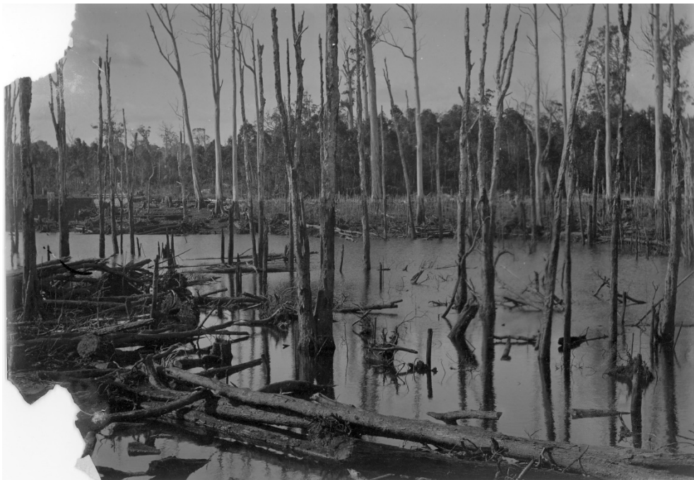
The Waratah Dam from within the impoundment, looking towards the dam wall, wooden weir and concrete spillway. Many trees have now died. The photo was probably taken to illustrate a particularly dry period at the mine. Photo courtesy of Liz Harris, Longford.
