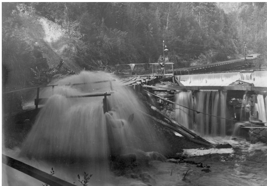
The Ringtail Flume discharging flood water into the Waratah River, 1906. JH Robinson photo courtesy of the late Nancy Gillard.
