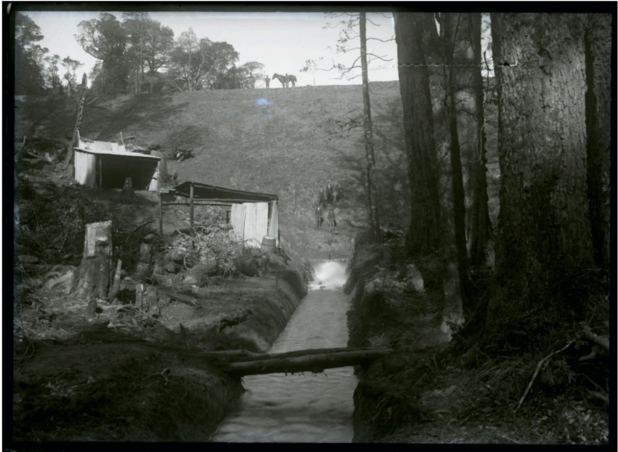
The outlet of the Magnet no.2 Dam below the dam wall, with water being released through a valve into a water race that emptied into a storage tank on a hill above the Magnet Silver Mining Company Power Station. Note that this dam had no spillway.
