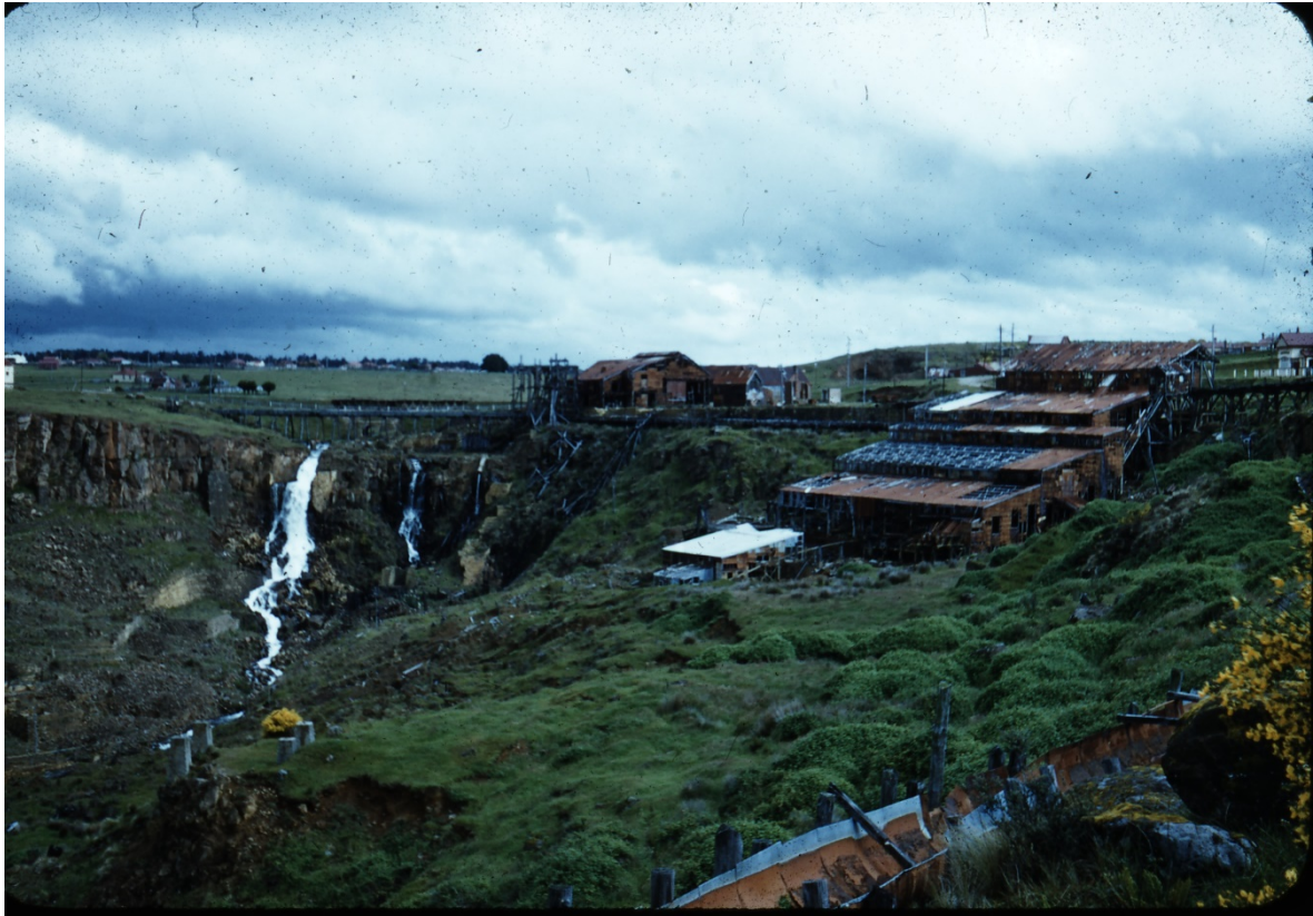
Waratah in the 1960s, after abandonment of the power station. The wooden flume remains over the Waratah River, but the metal flume (foreground) to the power station is decrepit.
