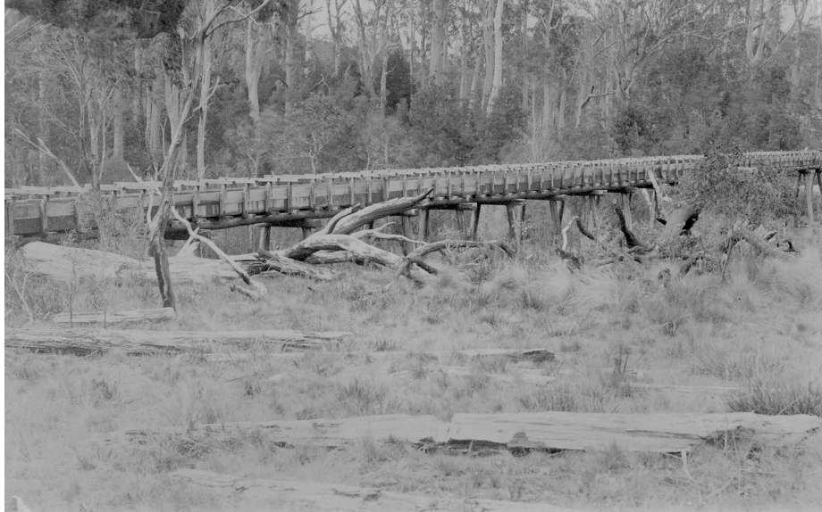
The Fosse Flume bringing water 6km from the Fosse River under Mount Pearse into the Fill 'em Dam (Bischoff Reservoir). Photo courtesy of Liz Harris, Longford.
