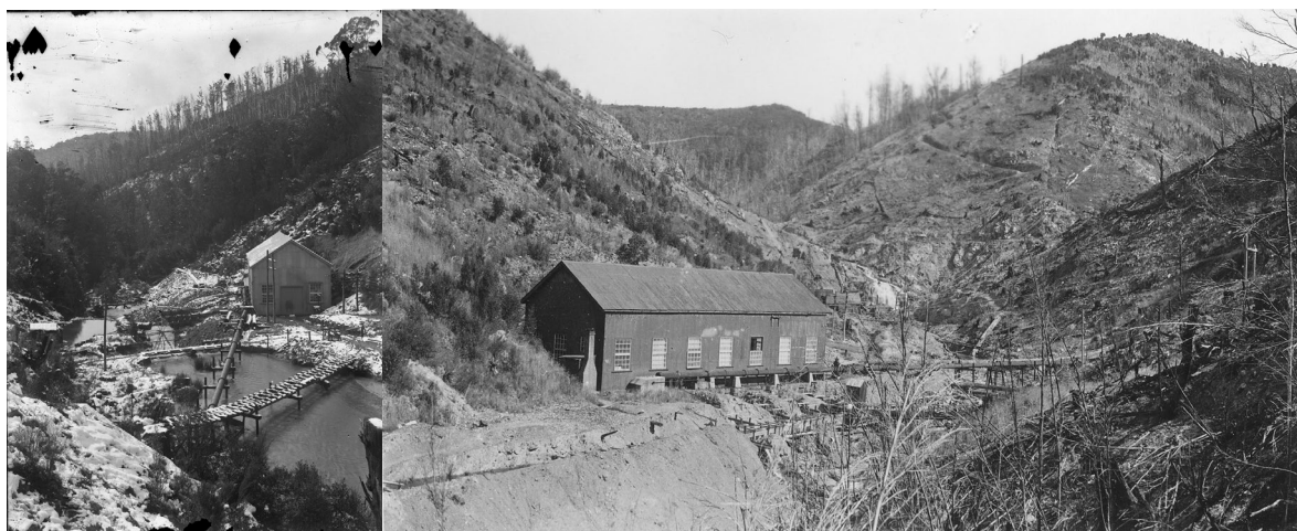
The Mount Bischoff Co Power Station in the Ringtail Gully, Waratah River, showing the water pipeline from the Black Tank crossing the river and entering the building. JH Robinson photos courtesy of TMAG and the late Nancy Gillard respectively.
