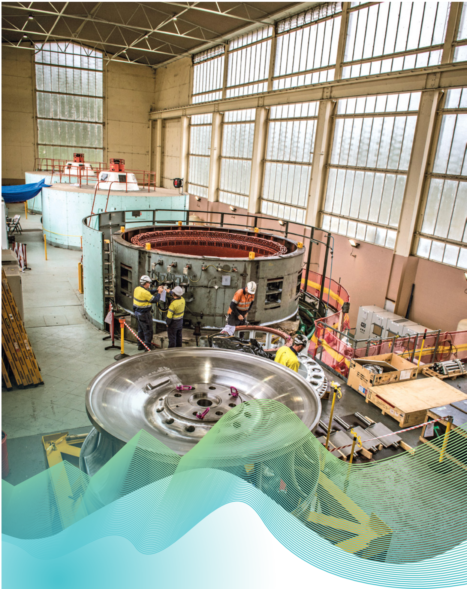
Above: Refurbishment works being undertaken at Wayatinah Power Station
