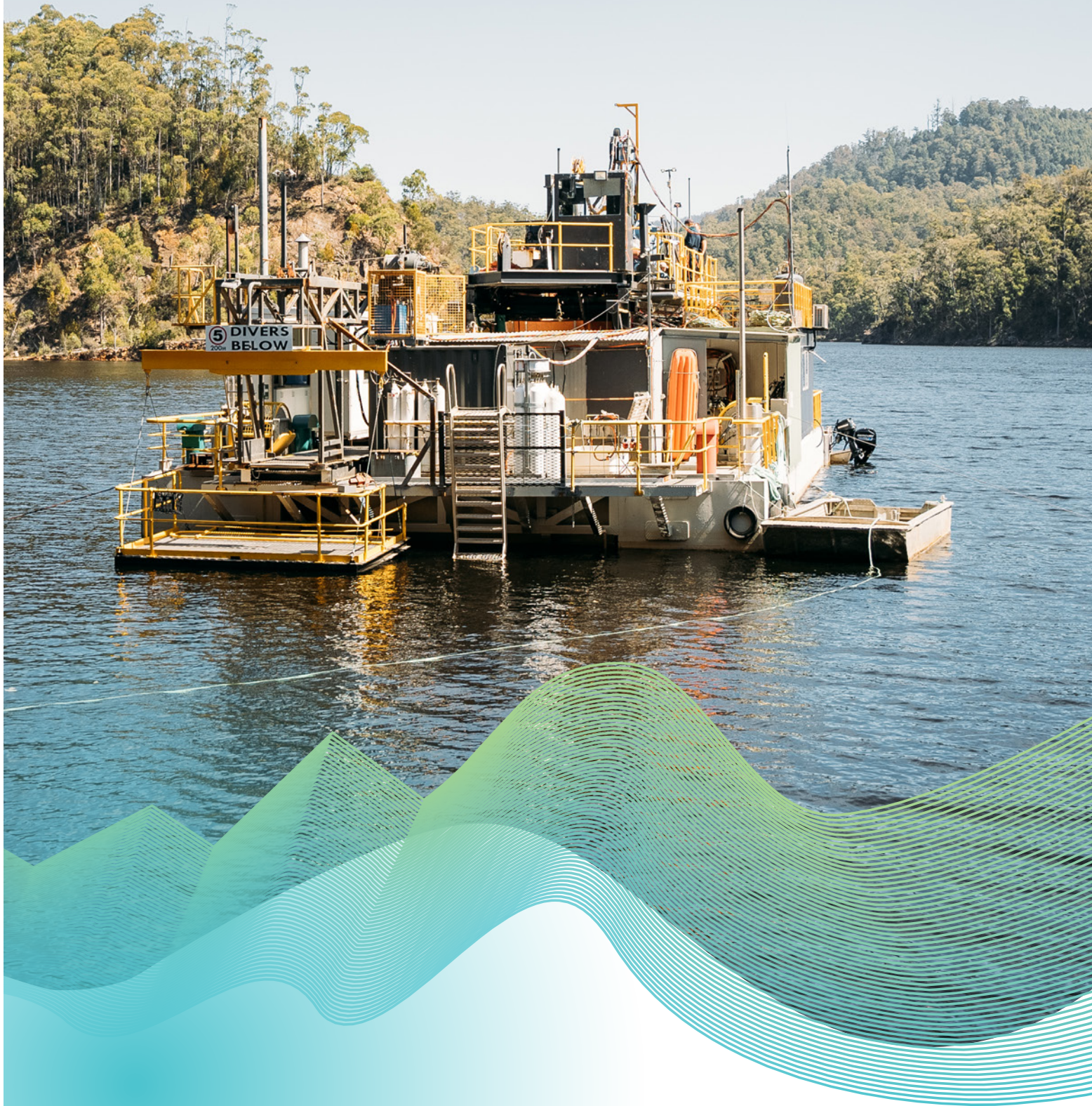
Above: Diving barge at Lake Cethana
