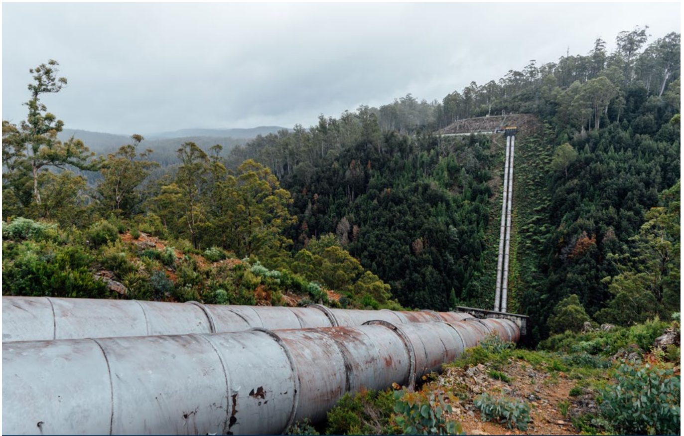
Mossy Marsh siphon at the Tarraleah canals
