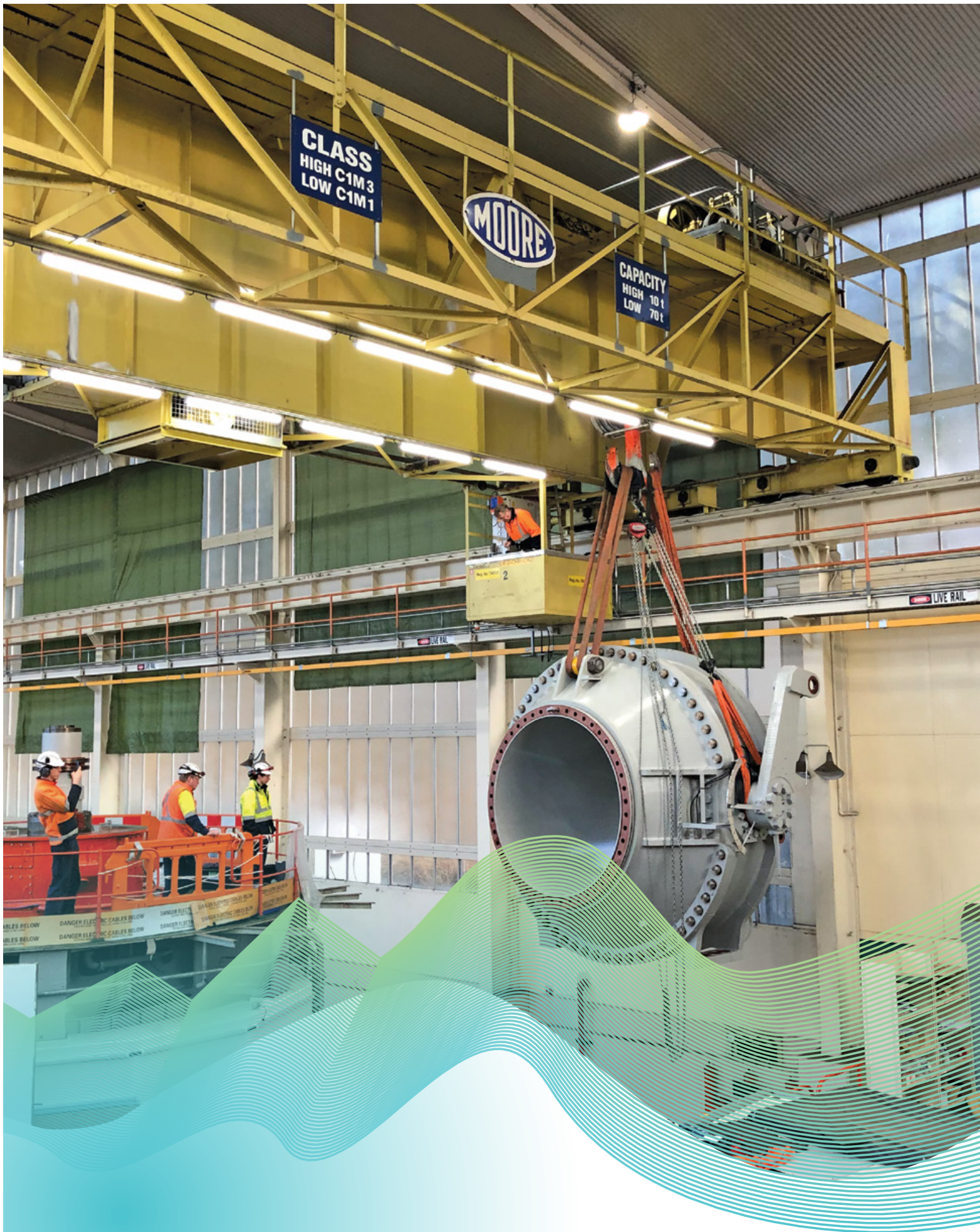
Above: Liapootah Power Station main inlet valve No. 3 installation
