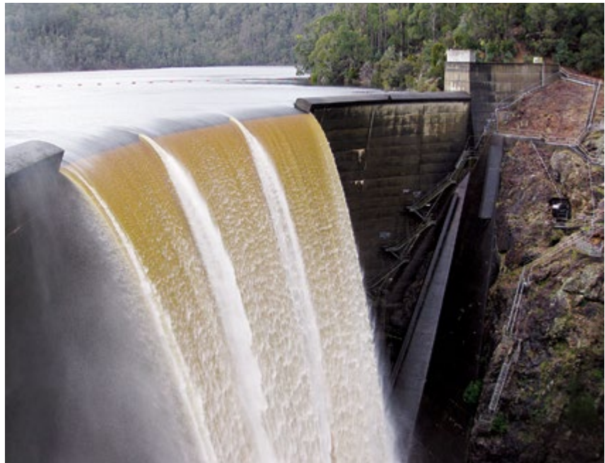
Spill at Devils Gate Dam
