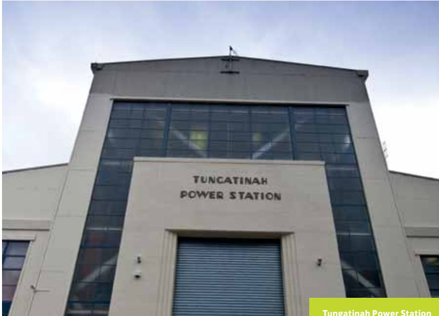
Tungatinah Power Station
