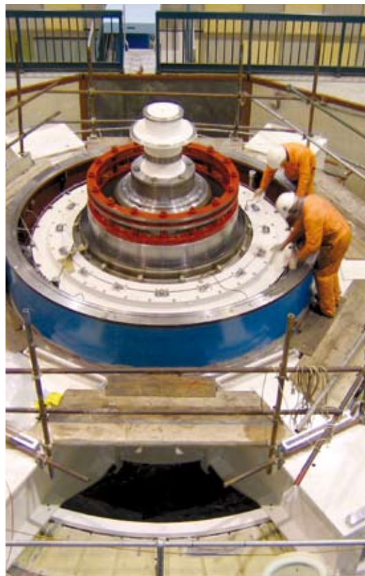
Gordon Power Station refurbishment
