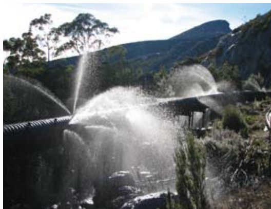
Woodstave pipeline at Lake Margaret
