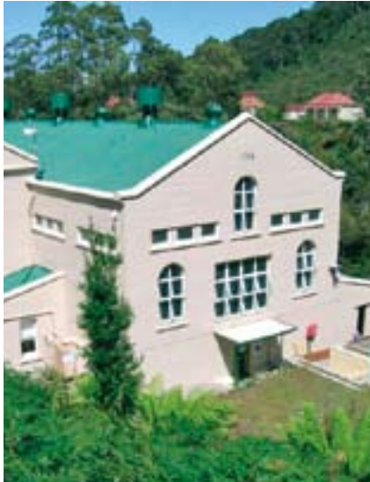
Lake Margaret Power Station
