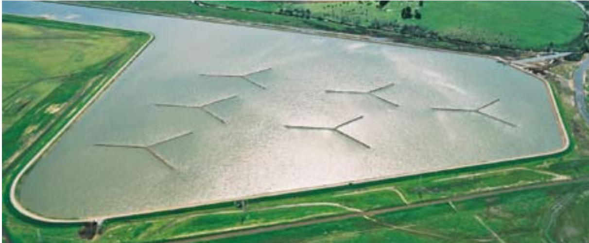
Poatina Re-regulation Storage with wind baffles integrated to minimise turbidity
