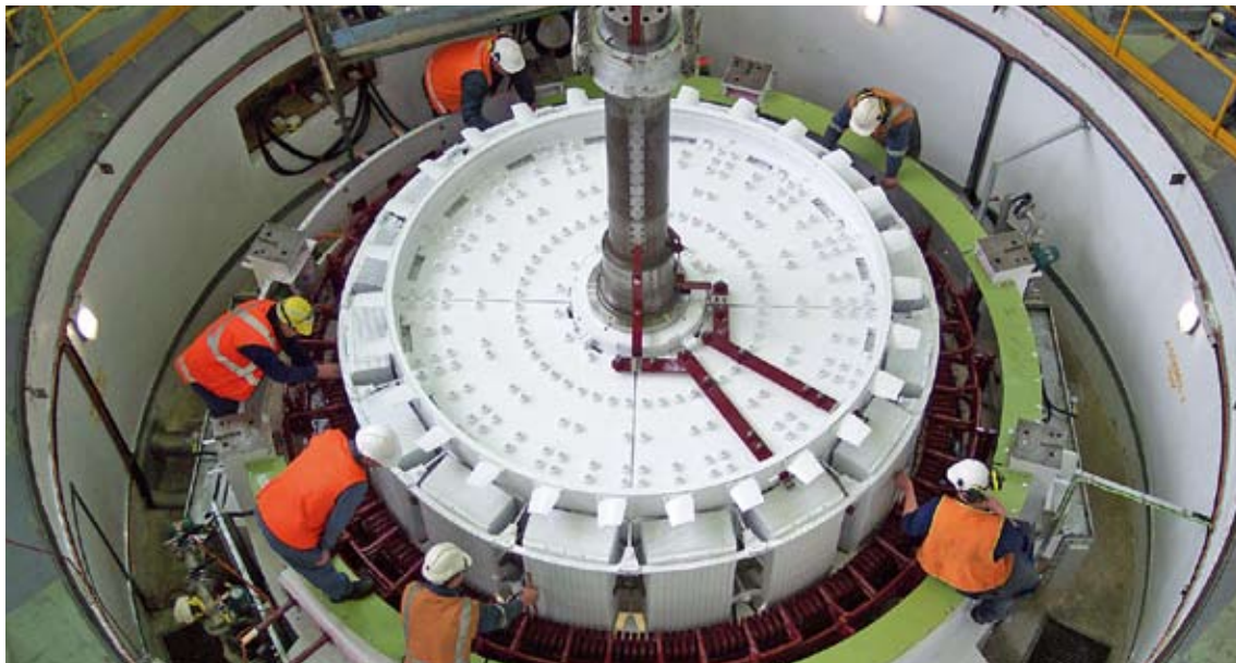
Work on hydro generation assets at Trevallyn Power Station
