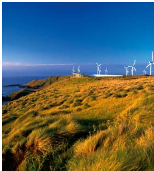
Woolnorth Wind Farm
